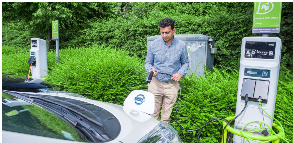
The Campus has expanded its provision for electric vehicles
